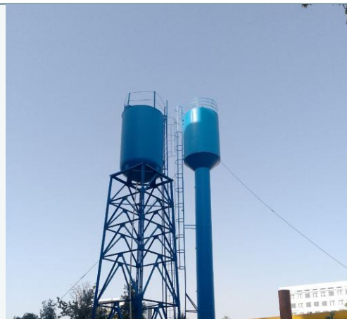
Photo 2. Water storage facility
