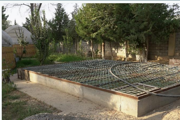
Photo 5. Wastewater treatment facility
