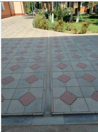
Photo 7. Green areas irrigated by recycled water
