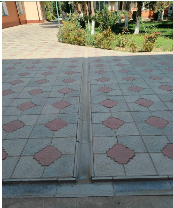
A4. Drainage channels and spring-water route
