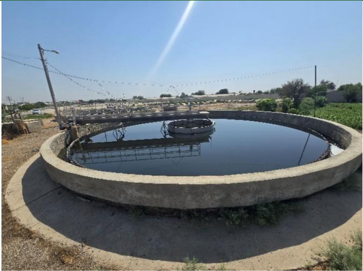
A3. Wastewater treatment facility
