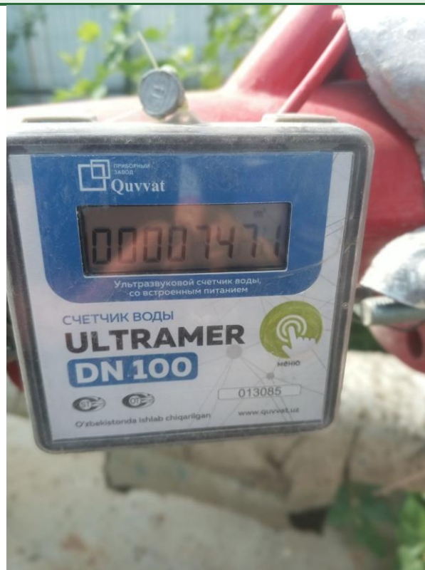
A10. Pollution-prevention infrastructure
