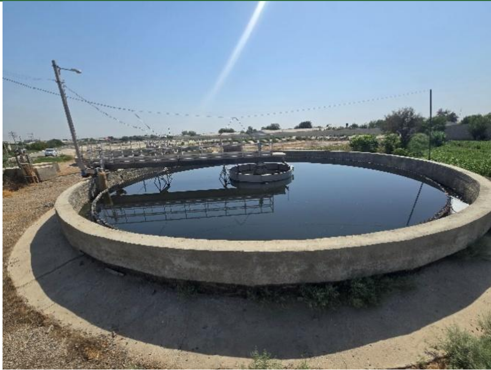
Photo evidence - Termez city wastewater treatment facility
