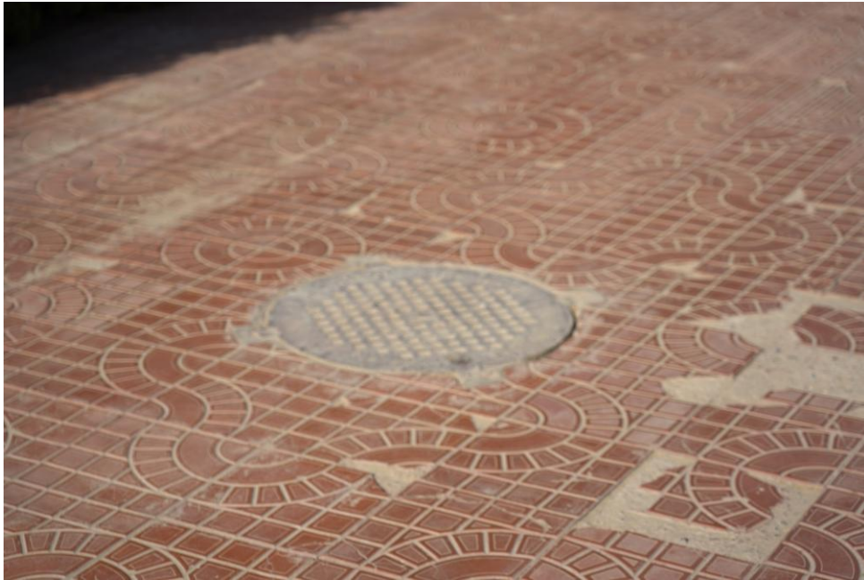
A5. Inspection chamber
