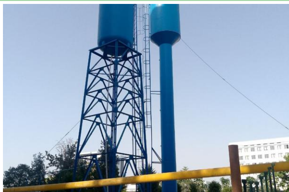
Water tower serving campus supply infrastructure.
