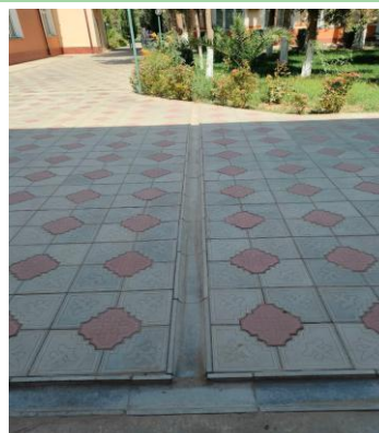
Controlled water flow and collection point inspected during field activities
