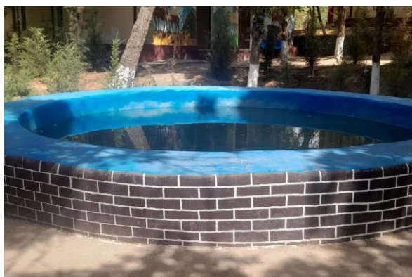
Rainwater-harvesting reservoir at a TerSU site.
