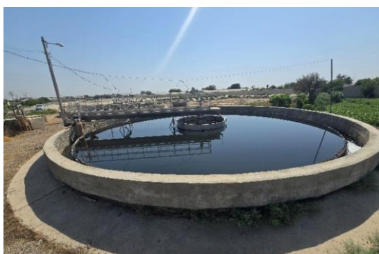
Wastewater-treatment facility serving the recycling chain.
