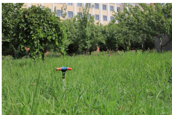
Water-saving sprinkler equipment in operation.
