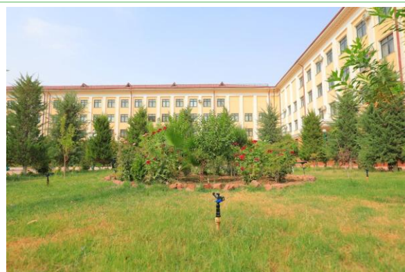
Green campus irrigation using water-saving equipment.
