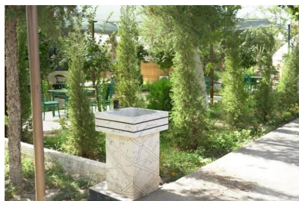
External clean-water distribution point.
